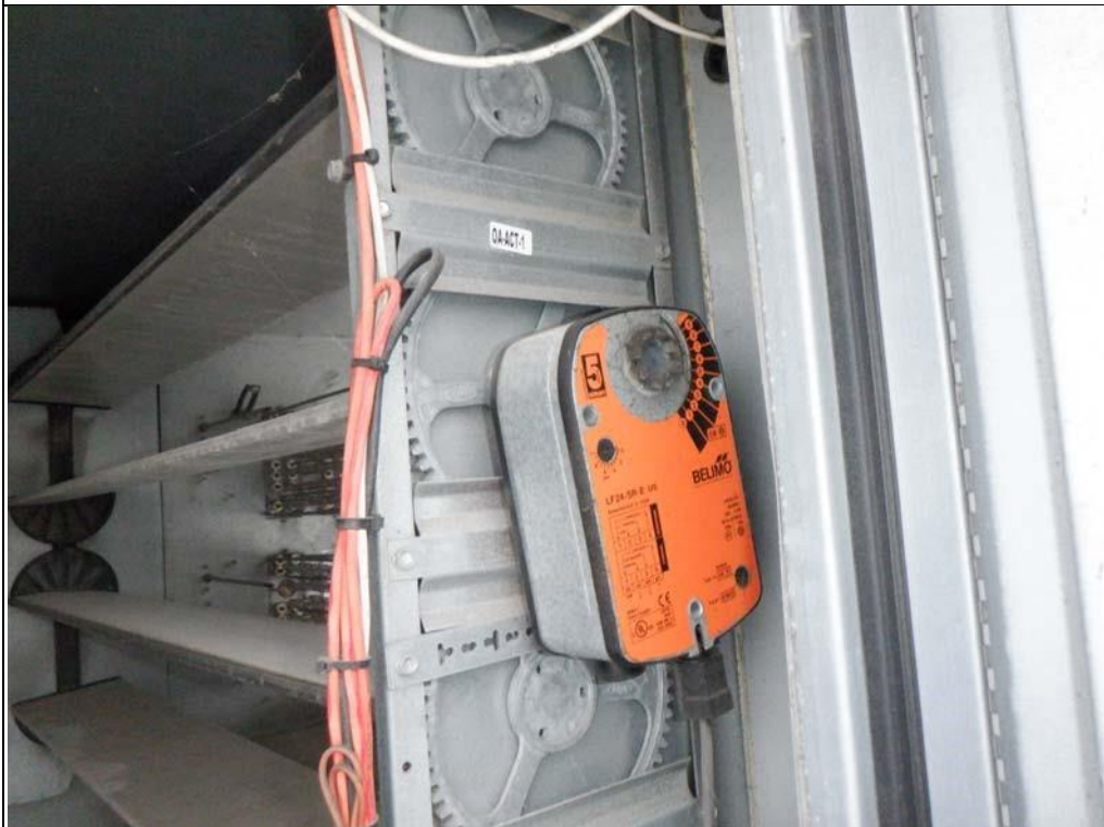
Servomoteur de registre, 35 in-lb [4 Nm], Ressort de rappel, AC/DC 24 V, 2...10 V, BELIMO LF24-SR-E US.
