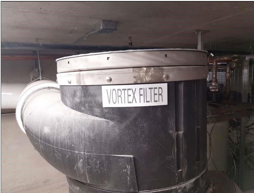
Filtre Vortex WFF300 ou WNR 430 RMS Rainwater management solutions.
