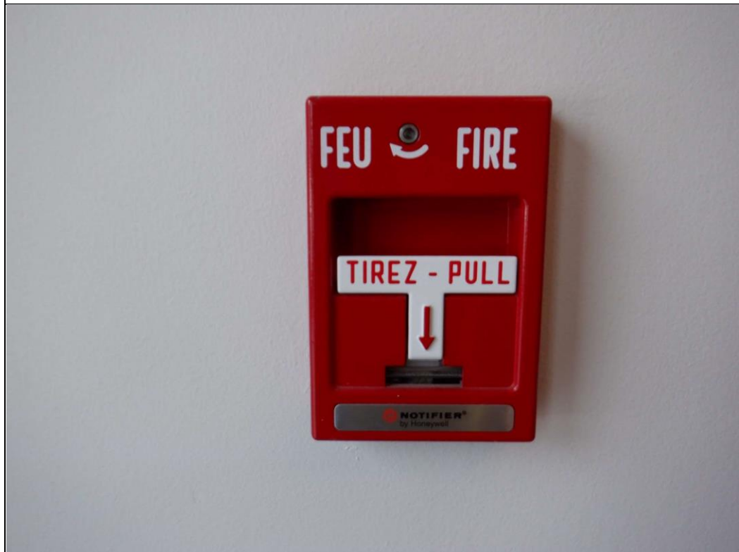
Station manuelle d'alarme incendie notifier by honeywell n-mps-sa / sac
