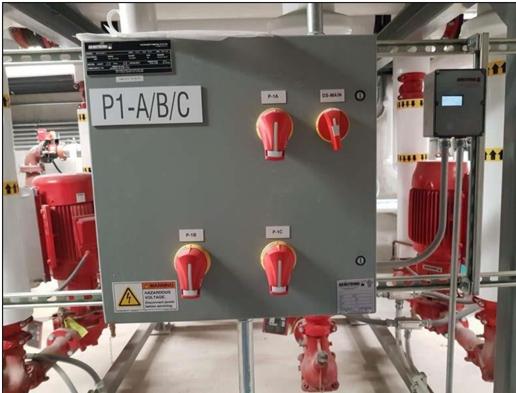
Panneau packaged pumping system ARMSTRONG CSTNMP P04740-01 EIC-01.
