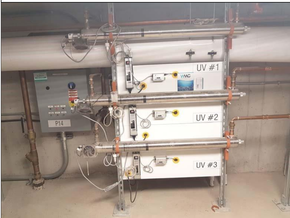
UV Dynamics 20GPM Classe "A" UVD20.40C UV Dynamics 20.40C.
