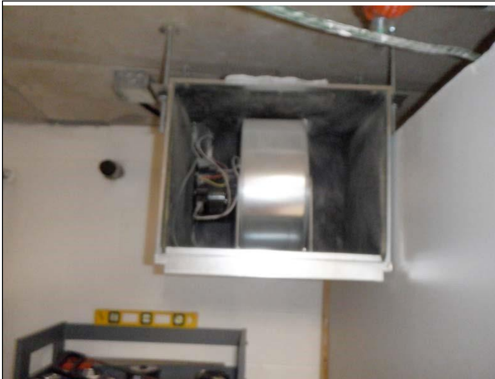
TF-P1.2 Ventilateur GREENHECK SP-A780-00.
