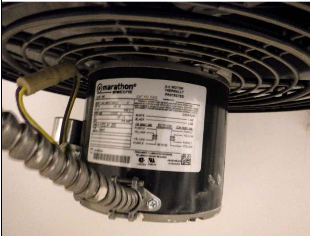
Moteur 1/6 Hp, 115, 48Y FR., 3 PH, 1075 Rpm, TEAO Marathon-Motors.com X306.
