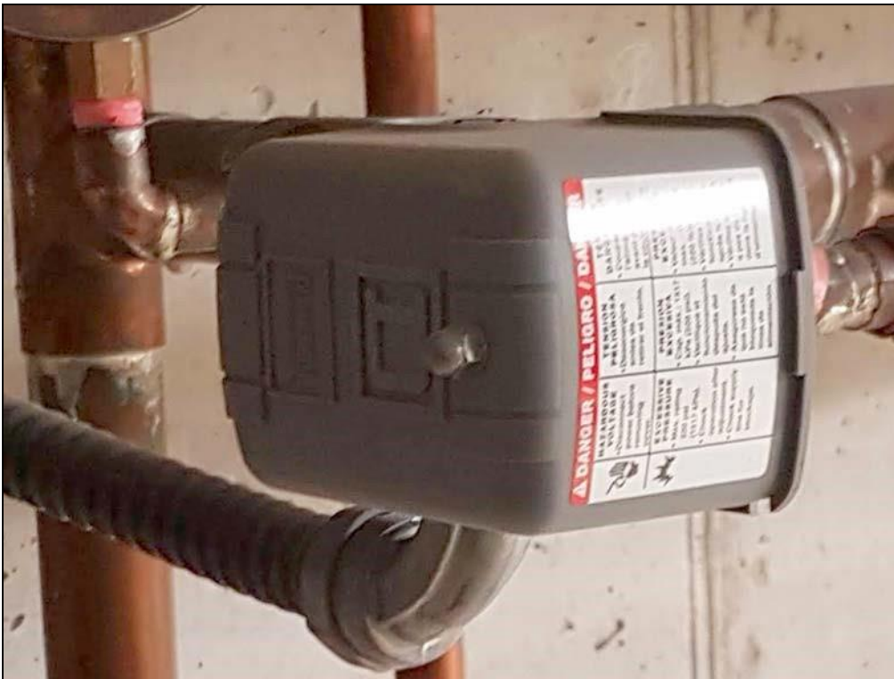
Pompe Pression d'eau 40-60 PSI Square D by Schneider Electric.
