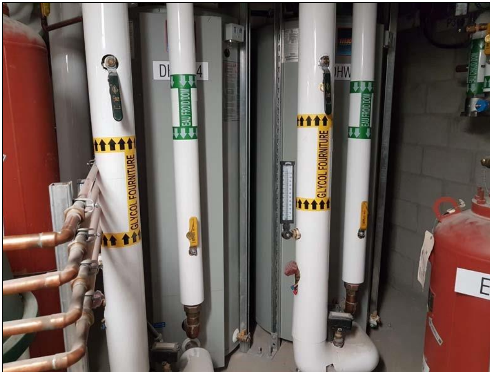
DHWT3 et 4 Chauffe-eau indirect instantané Turbomax 109 Thermo 2000.
